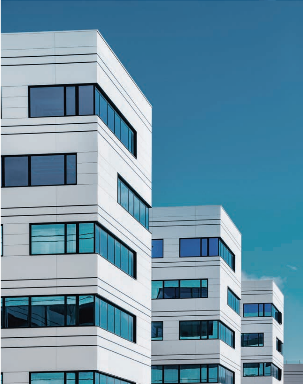
CHC MONTLÉGIA HOSPITAL, Liège, (Belgium)
