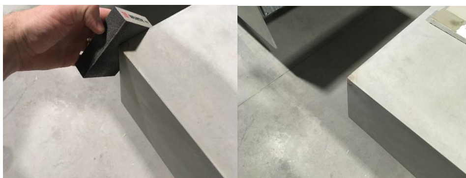
Photo: Example of additional sanding of the repaired area and its final appearance.
